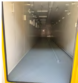
7. Insulation Installation Stage
