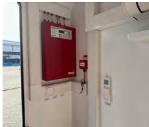
5. Electrical Installation stage (before testing)
